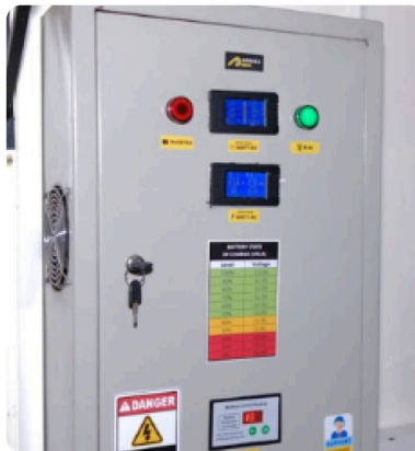
Instalasi Panel Surya
